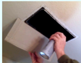
Spray inside of ceiling box flat black.
