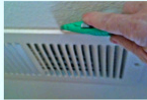
Remove old paint and caulking around vent
